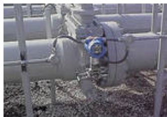
Plate 2: Flow Computer with Orifice Meter
